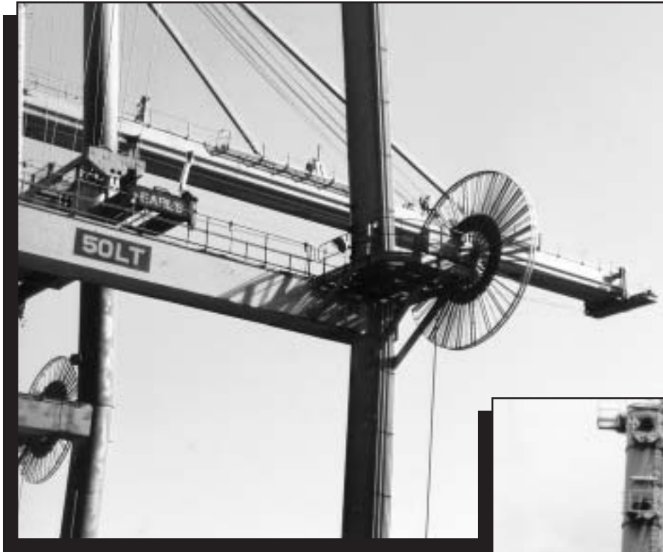
Container Crane To retrieve 1100 feet of #2 AWG, 3 conductor, type SHD-GC-5 KV high voltage cable.
