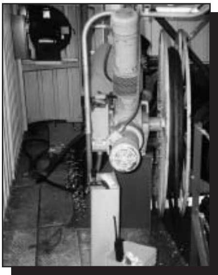
Container Spreader To lift 130 feet of #12 AWG, 36 conductor, type SO cable.
